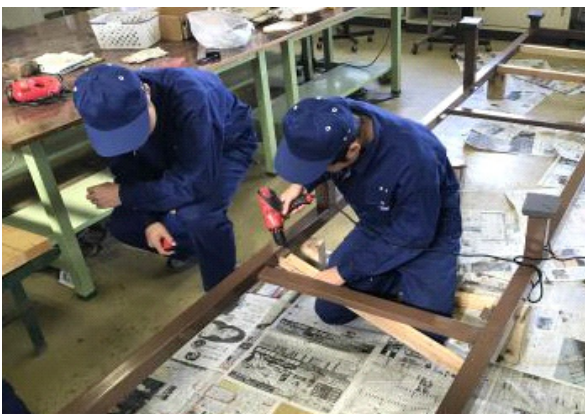
Photo 56: Building the ramp framework
