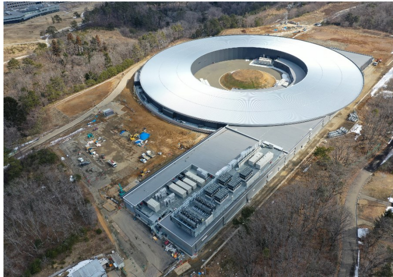
Next-generation synchrotron radiation facility (under construction)
