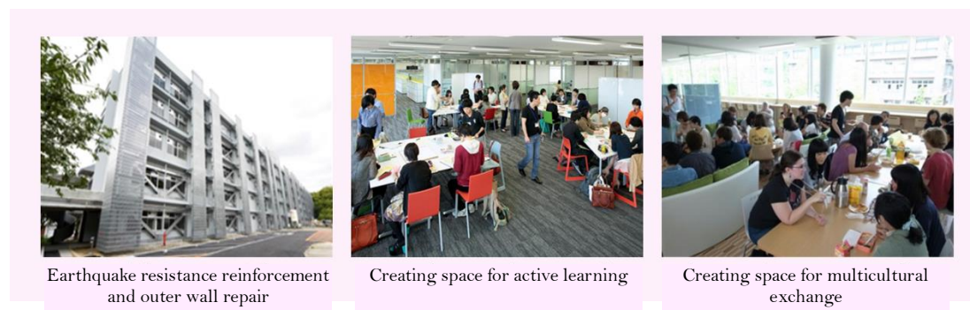
■ Figure 2-4-12/ Examples of Facility Improvement for Securing Safe and Secure Education/Research Environment and Function Enhancement of National Universities, etc. ■
