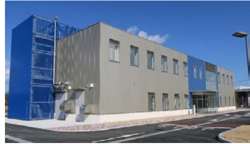
International Collaborative Research Building Collaborative Laboratories for Advanced Decommissioning Science Source: JAEA
