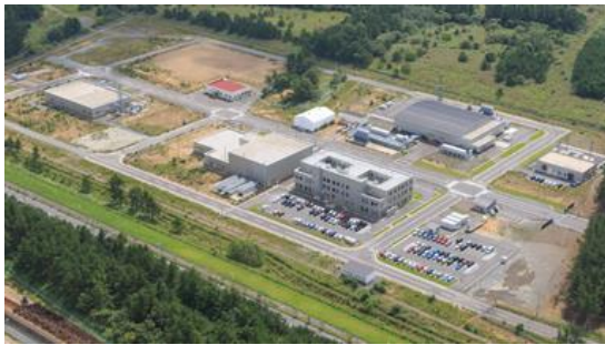
International Fusion Energy Research Center (Rokkasho Village, Aomori Prefecture)
