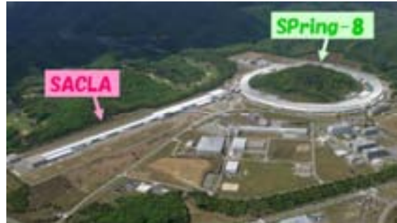
Super Photon ring-8 GeV (SPring-8) and X-ray free electron laser facility (SACLA) (The long shaped building on the left is SACLA. The round building on the right is Spring-8.)
