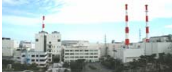
Tokai reprocessing facilities Photo: Japan Atomic Energy Agency
