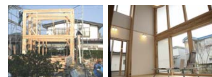
Rigid-frame wooden house with glued-in hardwood dowels
